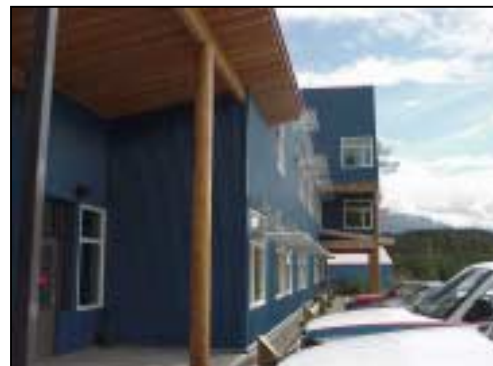
A view of the Extensive Use of Overhangs on the South Side of the Building
