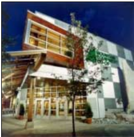
A central roof monitor daylights the Mountain Equipment Co-op store to create a superior shopping environment.
