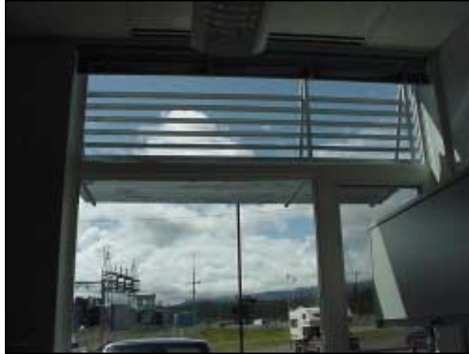
A View of Exterior Louvers From the Inside
