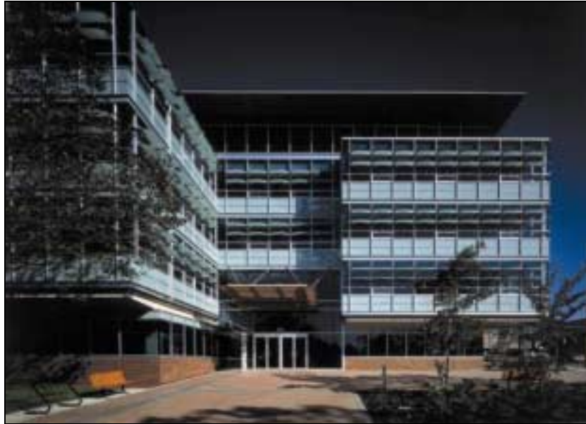
The Revenue Canada Burnaby-Fraser Tax Services Building
