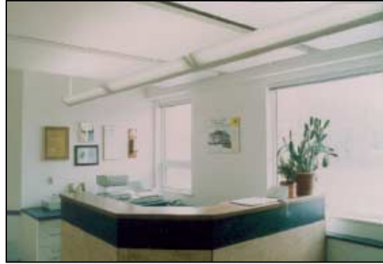
Radiant Heating and Cooling Panels
