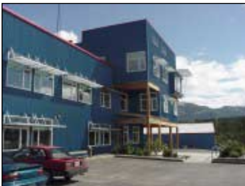
A view of the Extensive Use of Overhangs on the South Side of the Building
