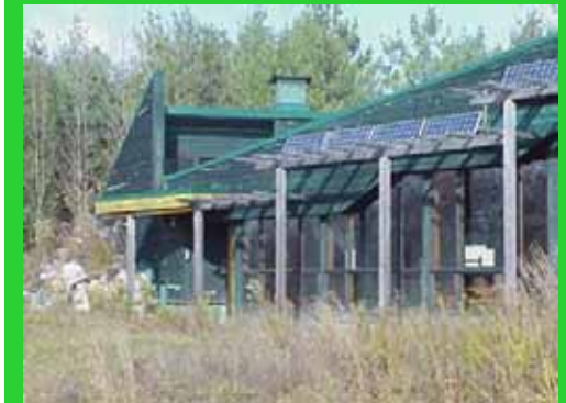
All of the wood cladding at the YMCA Environmental Learning Center, Paradise Lake, Ontario was salvaged from the demolition of an existing building.
