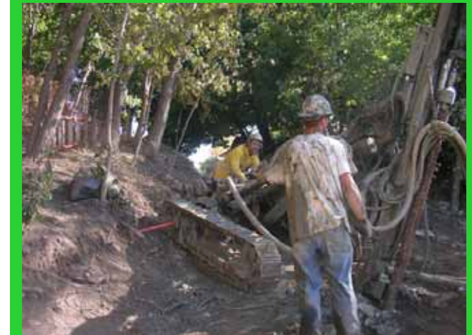
Difficult foundations for a tree, sloped site for the Grand House Student Cooperative in Cambridge, Ontario, Canada
