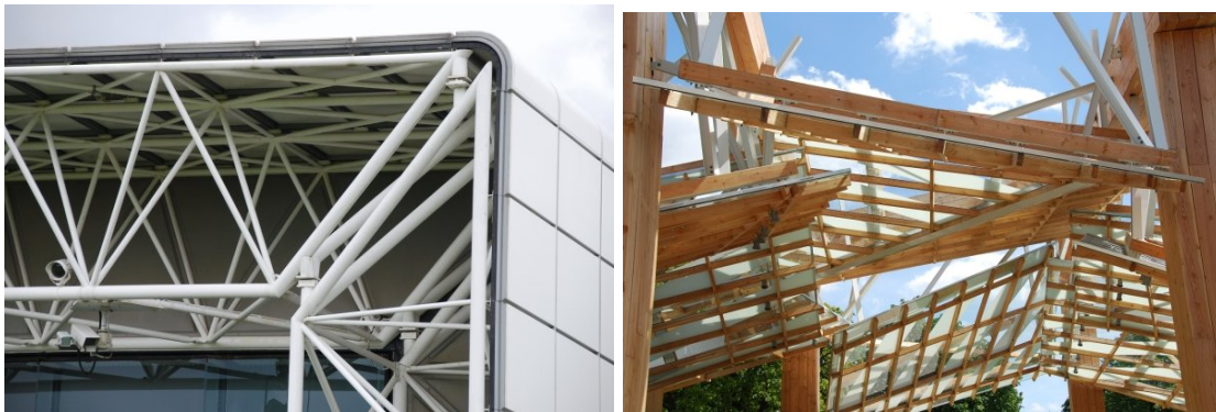
Fig 1: Foster's Sainsbury Center (1977) and Gehry's Serpentine Pavilion (2008) both require that the Architect understands structure and construction detailing.
