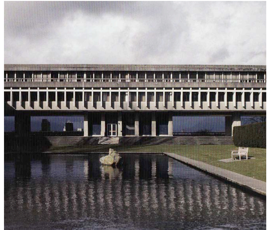
(Fig. 6.) The arcades opening themselves to frame views of the mountains beyond
