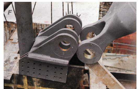
Pompidou Center, joint detail
