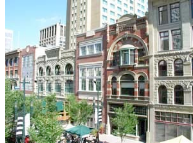
Architectural Details of the Historic Facade
