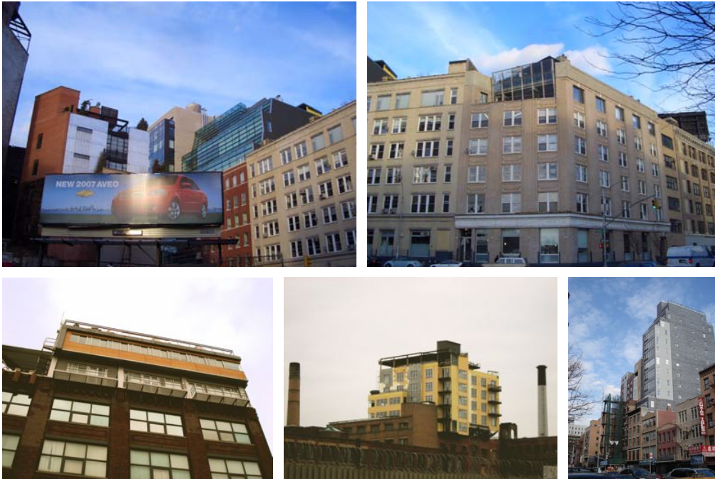
Figure 6. Built Examples, New York. Clockwise from top left, Canal and Greenwich Sts (2), Bowery and Spring, DUMBO (2)
