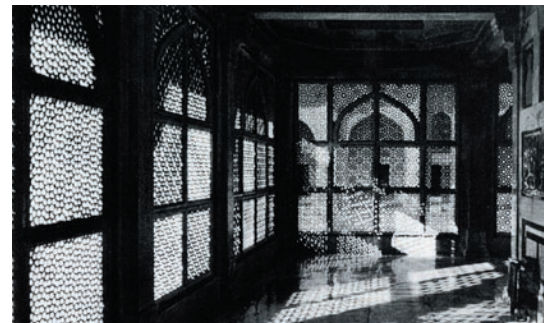
Mogul screens act as sophisticated shading devices in Indian structures, creating dramatic plays of light within spaces (Behling, 1996, 117)
