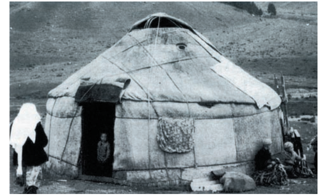
The yurt, a lightweight, lattice-structured structure that can be contracted for transportation, found in varying regions, but typically in arctic climates (Behling, 1996, 49)
