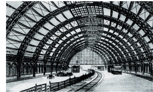
A comparison of a greenhouse and railway station, both informed by the architectural developments brought by the Crystal Palace (Minter, 1990, 13), (Behling, 1996, 141)
