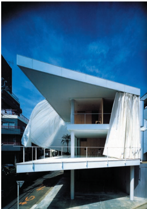
Curtain Wall House, Itabashi-Ku, Tokyo (Ban, 2005, 50)
