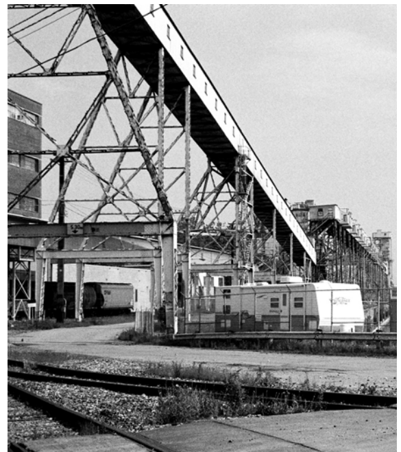
Fig. 13: Skeletal structures supporting elevated galleries leading to marine towers in the background. Photo by author, 2006.
