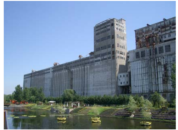
Fig. 9: 2006 photo of the 'B-1 Annex', with temporary landscape exhibit in the Lachine Canal basin. Photo by author.
