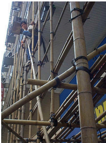
ILL.02 - bamboo scaffolding
