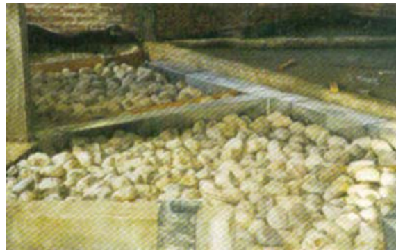
Greenhouse and rockbed systems in the Bariloche Ecohouse by Manuel Fuentes xiii
