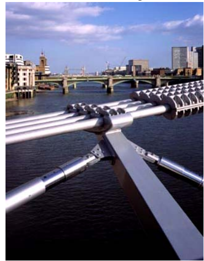
Millennium Bridge Detail
