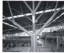
1.12 Stuttgart Airport Roof using tubular column 'trees' — see also Colour Plate 9 (architect: Von Gerkan Marg & Partners)
