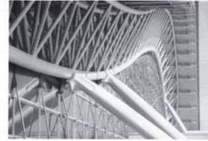
1.13 Tubular trusses at Kansai Airport, Japan (architect: Renzo Piano Workshop)
