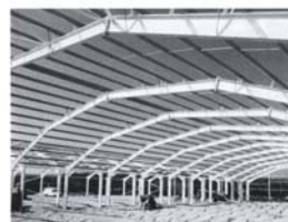
3.11 Long-span portal frame used to create an arch structure
