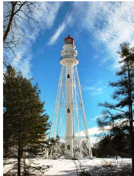
Rawley Point Lighthouse: Steel Skeleton Tower Construction
