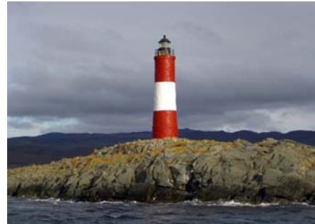
Les Eclarieus Lighthouse: Reinforced Concrete Construction
