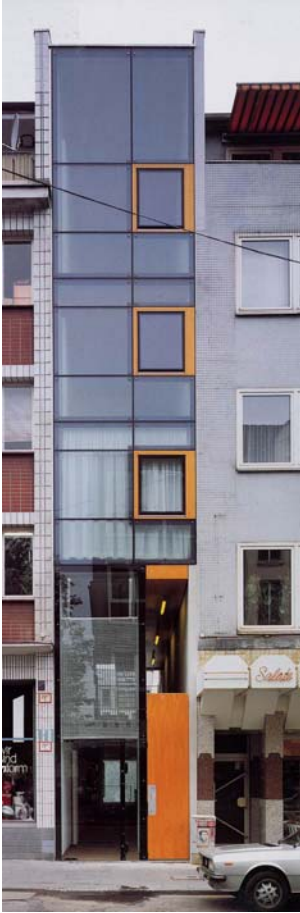
4. Apartment building in Cologne, Germany
