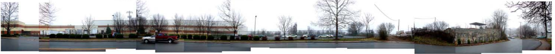
View north from site to warehouse and cement factory across Carlton Avenue
