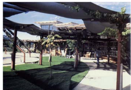
Figure 8.2 South trellis and shading devices on the south facade of the Real Goods Solar Living Center. (Margot Kelly McDonald)
