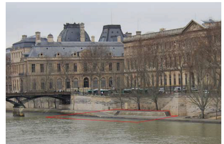
Figure 7: Site Bounds looking at both retaining wall and bridge
