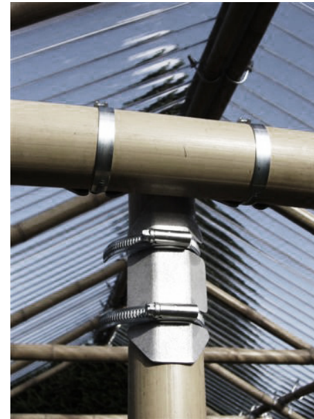
Fig. 12: Bambootix System Typical Detailing
