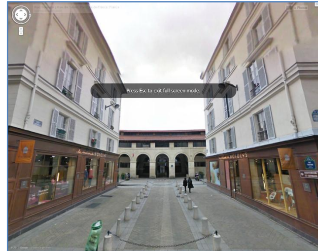
1 The existing building on our site on the left; its twin on the right (source: maps.google.com)
