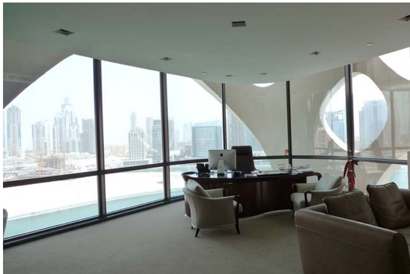
Figure 8: A view of an office interior showing the continuous nature of the floor to ceiling glazing that creates the inner layer of the double façade.
