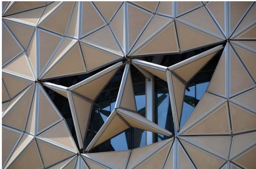
Figure 10: A view of one of the panels during construction showing three “umbrellas” in a fully open position. Once commissioned the action of the opening and closing will be consistent and follow the path of the sun allowing for a more open view during non-solar times.
