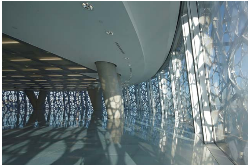
Figure 5: A view of the interior of one of the office floors showing the effect of the geometric screening on the interior. Not all direct sunlight is blocked in order to preserve significant views from the tower. Photo courtesy Ateliers Jean Nouvel and CSCEC.
