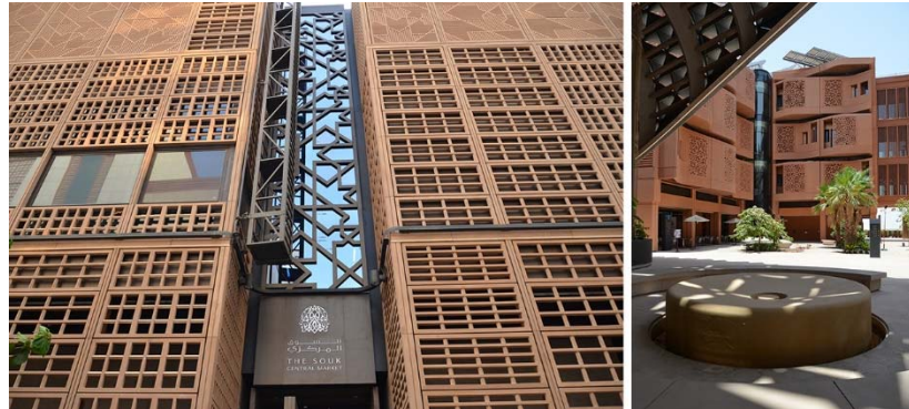
Figure 2: Two modern interpretations of the Islamic mashrabiya. Left, The Souk and right, Masdar City, both projects located in Abu Dhabi, UAE and both from the offices of Foster + Partners.
