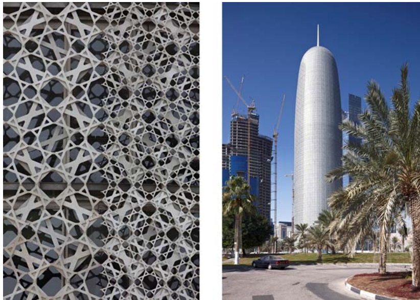
Figure 4: A view of the variations in the density of the screen pattern on the Doha Tower. The variation in density to achieve different screening results is achieved by the simple layering of the prefabricated components. Photos courtesy Ateliers Jean Nouvel and CSCEC.
