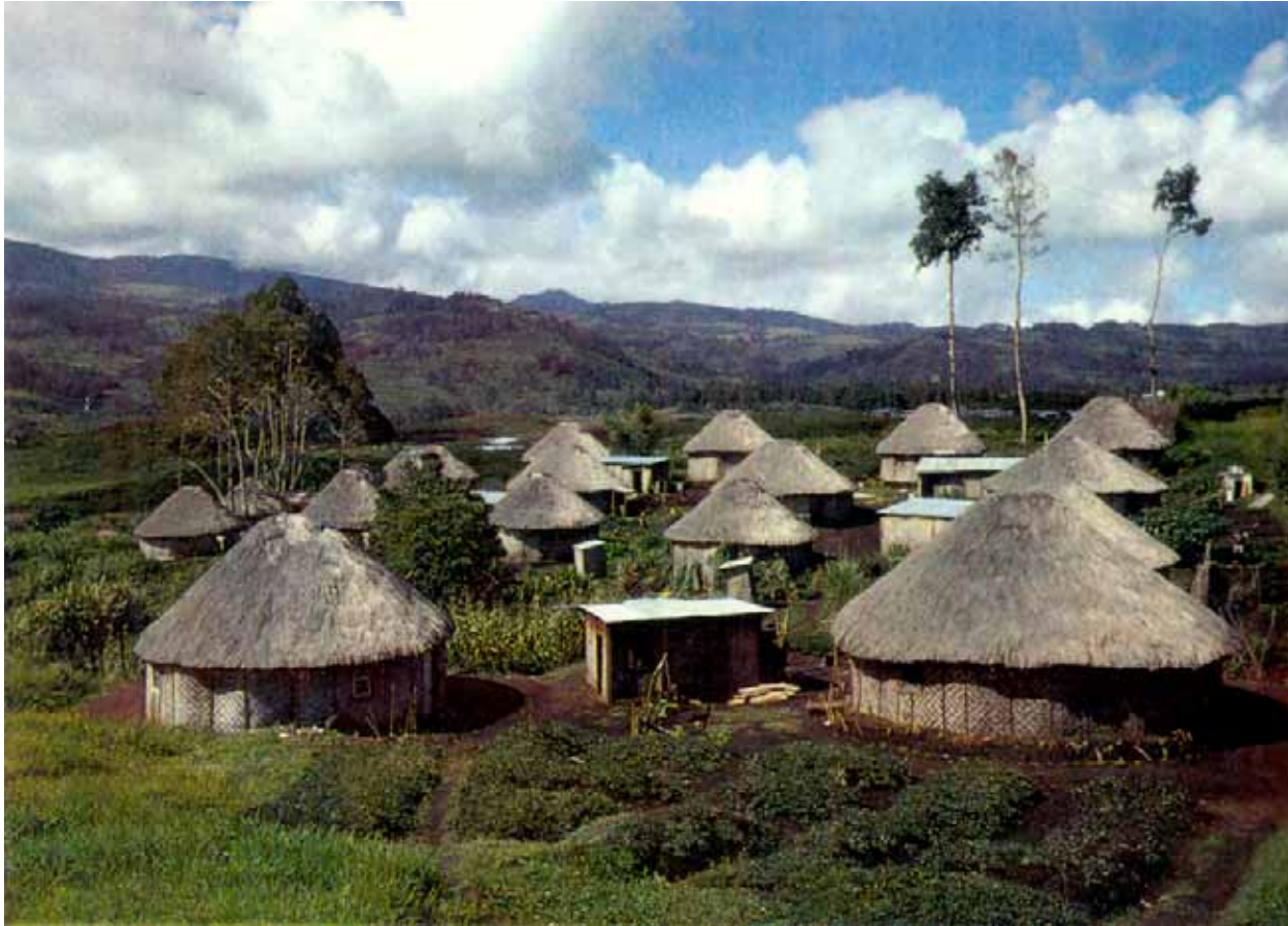
Conical thatched grass roofs top circular dwellings built with interlaced fiber siding , Village in New Guinea
