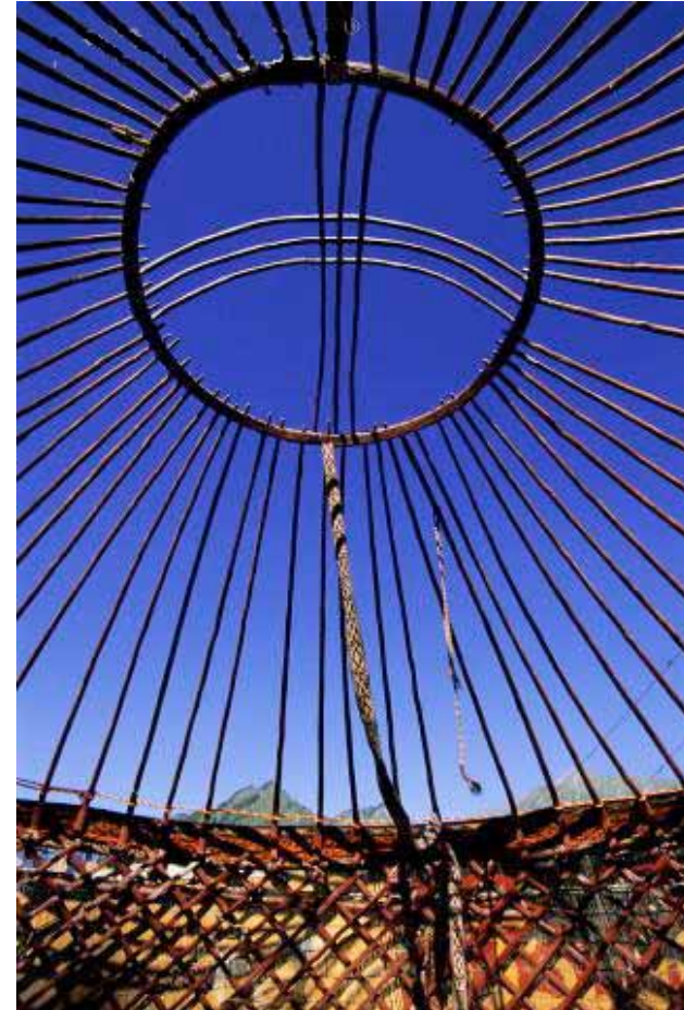
Mongolian YURT with collapsible “pantograph” side walls, and felt mat covering.
