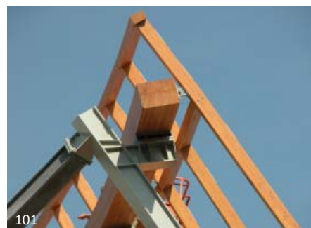
Here galvanized steel members are mixed with zinc painted grey steel. It was decided not to galvanize some of the members due to the chance of deformation in the hot zinc bath and potential stress release of the welds.
