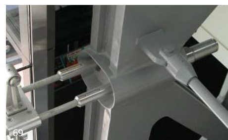
Fig. 4.2B It is easy to see that this detail relies on a high level of finishing - including grinding and contouring of the welds, to achieve its Form, Fit and Finish.
