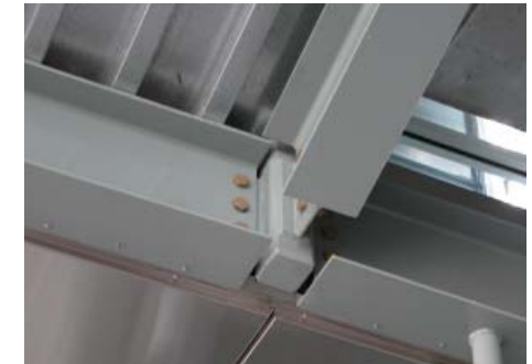
Fig. 3.5B This exposed bolted connection is tightly designed and demonstrates uniformity in the joint gaps.
