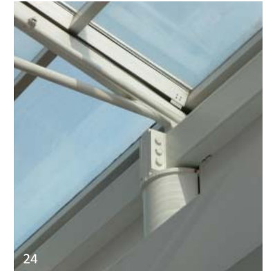
Pierre Elliott Trudeau Airport, Montreal: The trusses supporting this skylight are quite characteristic of AESS 2 type steel. The viewing distance is over 6 metres but the design wishes to use something more than a standard joist or truss. The detailing is simple, and the viewer is not close enough to see the texture of the connection, only the form of the truss.
