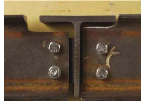
Fig. 3.5A Joint gap minimized. The gaps on the left are standard structural steel. On the right sized for AESS. Courtesy AISC
