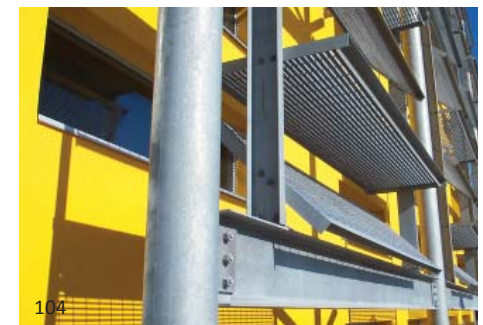
Galvanizing is very popular as a "finish" but remember that its basic purpose is as a corrosion prevention coating. The nature of the finish will not be consistent from batch to batch.
