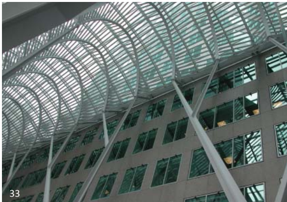
33 BCE Place in Toronto by Spanish Architect Santiago Calatrava uses AESS 4 quality fabrication and finish on the lower portion of the tree supports in the Galleria space. All of the members use welded connections with a hand smooth finish and no apparent blemishes. Given the articulation and complicated geometry, tolerances for this structure were even less than one half standard fabrication. The “canoes” that form the support for the skylight are well above view level and use a combination of welding and bolting.
