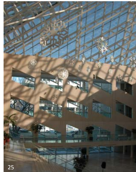
Edmonton City Hall: The trusses that support the pyramidal glass roof are created using square HSS sections. The viewing distance varies, but is typically greater than 6 metres, even from the upper levels. An up close inspection reveals many inconsistencies that are reasonable to leave “as is” due to the view distance. The extra expense to fill, grind and carefully align the members would be lost on users of the building.
