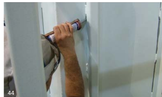
Fig. 1.3 filling between the intermittent welds to give a continuous weld appearance.
