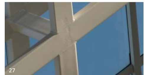
Edmonton City Hall: The trusses that support the pyramidal glass roof are created using square HSS sections. The viewing distance varies, but is typically greater than 6 metres, even from the upper levels. An up close inspection reveals many inconsistencies that are reasonable to leave “as is” due to the view distance. The extra expense to fill, grind and carefully align the members would be lost on users of the building.
