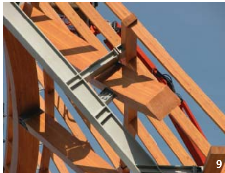
Composite structural systems require higher levels of coordination and that the tolerances and construction practices of the other material be taken into account.
