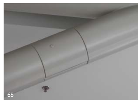
Fig. 3.6A Pictured is a cover plate over a hidden bolted connection. The appearance of a completely welded structure is kept, but erection simplified.
