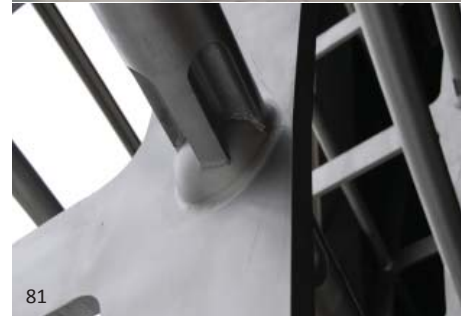
The Chinese National Theatre uses large plate steel members to create its trusses. These in turn are braced by solid rods that use a half sphere to manipulate the curve of the connection. The form, fit and finish on the project are very high. This was undoubtedly the result of significant coordination and close supervision of the work.
