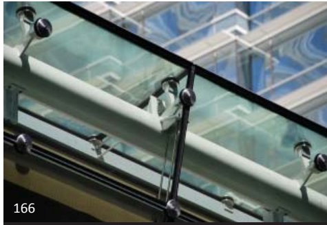
166 Spider connectors are used to connect this mullionless glass to a tubular steel frame at the top of the expanse of window of this Las Vegas Hotel lobby. The coordination for this detail is extremely tight, with little room for discrepancy given the proximity of the steel tube to the inside face of the glass.
