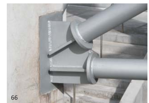
Fig. 3.6B This design used all welded connections, even for this anchoring detail of the truss to the base plate. Bolted connections were not desired.
