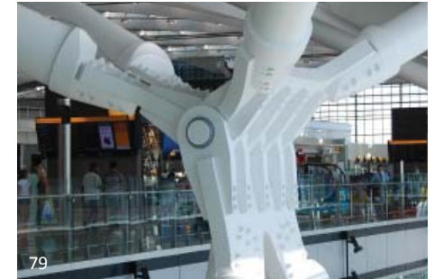
Complex geometry, odd angles and extremely heavy elements adds a cost premium to this project. The level of form, fit and finish on this project is exceptionally high. In the UK a high level of tradition of AESS has been established which has resulted in a highly skilled labour force.
