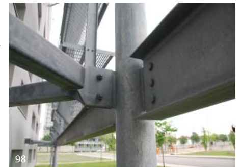
98 As can be seen in this galvanized exposed steel exterior shading system, a variety of finishes can be seen on the different hot dip galvanized members. This is to be expected in this sort of application.
