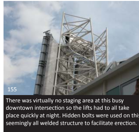
The erection that took place at this end of the building was extremely challenging as the crane operator was "below" the pieces he was erecting and the small staging area was bordered by hydro wires. It is not uncommon with such a small staging area and such complex geometry for it to take more than one attempt to fit a piece.
