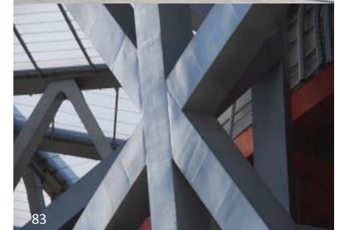
The scale and complexity of this welded project meant high cost premiums and additional fabrication and erection time. The project was additionally complicated as a result of fabrication and erection in China. There is far less AESS work that is routinely made a part of their construction so skilled labour can be an issue. The sections were created using plates and given varied lighting conditions many of the welds were visible. The overall aesthetic of the project could accommodate this level of texture.
