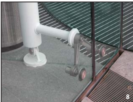
Specialty glazing systems require tighter tolerances and a higher level of FIT on a project.
