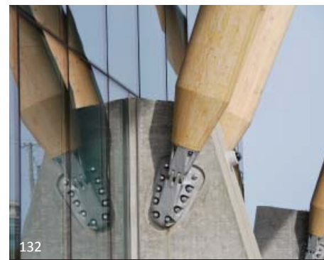
Custom castings are used to connect the timber columns to the concrete foundations.
