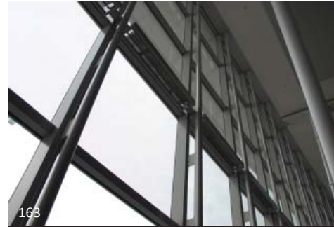
163 The AESS system illustrated here uses a specialized vertical truss like column formed from round HSS sections and plates, with holes cut into the plates to lighten the appearance of the system, to act as the lateral wind load support for this very tall expanse of glass at Pearson Airport. The thin profile of the steel appears as a simple extension of the curtain wall.
