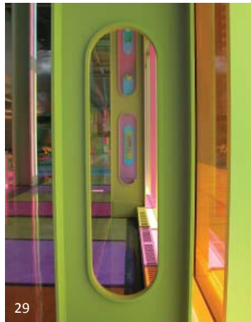
The Palais des Congrès in Montreal uses specialty W sections with trimmed cutouts. Although the steel is all painted grey, and intumescent coatings are used, the coloured light through the curtain wall gives additional texture to this expression of steel.
