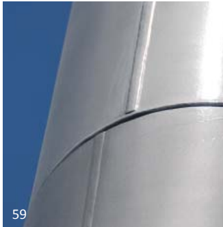
Fig. 3.3A The natural weld seams on these connecting HSS sections may have been better detailed if they had been aligned.
