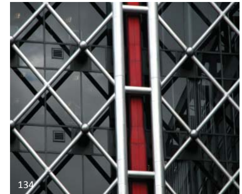
All of the primary connections on this project are fabricated from cast steel.
