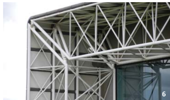
The Sainsbury Centre for the Performing Arts was designed and constructed by Norman Foster in 1977. The British High Tech movement brought exposed structural steel to the forefront of design, and with it an array of issues that had not been part of architectural discourse for more than a century. The project used round HSS members and a structure that was expressed on the exterior and interior of the building.
