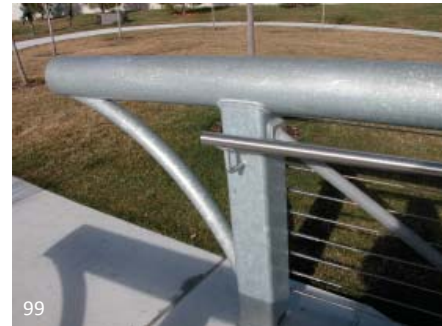
Seal welds have been used to connect the various components of this exterior galvanized steel feature railing. There is a large opening at the base of the square HSS post to allow any water that may enter the railing an opportunity to drain.
