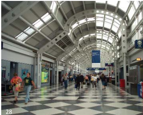
O'Hare International Airport in Chicago was the first airport to use AESS. Much of the steel is well within range of view and touch. A variety of steel shapes and connection types have been used. The complex nature of the sections and connections called for a tighter sizing tolerance and even finish application.
