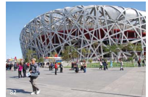
Complex geometry, odd angles and extremely heavy elements adds a cost premium to this project. The level of form, fit and finish on this project is exceptionally high. In the UK a high level of tradition of AESS has been established which has resulted in a highly skilled labour force.
