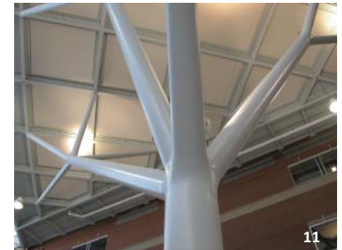
Two different steel trees. One created using W shapes to create a very textured appearance, the other using mechanical pipe and specialty casting and striving for a seamless appearance, using a high gloss finish. AESS specifications must be tailored to the overall design intentions of each individual project as they are all somewhat unique.
