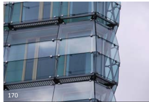
170 The steel supports for this double façade envelope use a system of clips to support the extra layer of glass. This alleviates issues of drilling of the glass and allows for better accommodation of differential movement between the systems.
