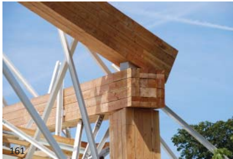
161 The heavy timber on this scupltural project is really "for show" as the main support system is all steel and the large square wood sections are used only to bulk out the form and provide a contrast with the steel used to support the glass.
