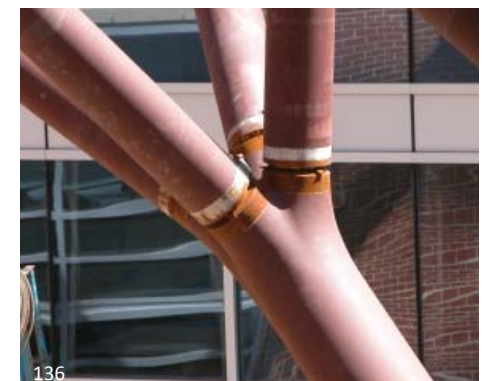
A large steel casting was used in this tree like structure to join several mechanical pipe sections. The joints were filled and sanded to conceal them.
