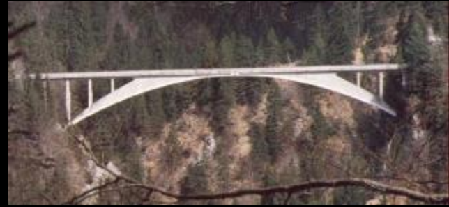
Salginatobel Bridge Schiers, Switzerland Robert Maillart 1930
