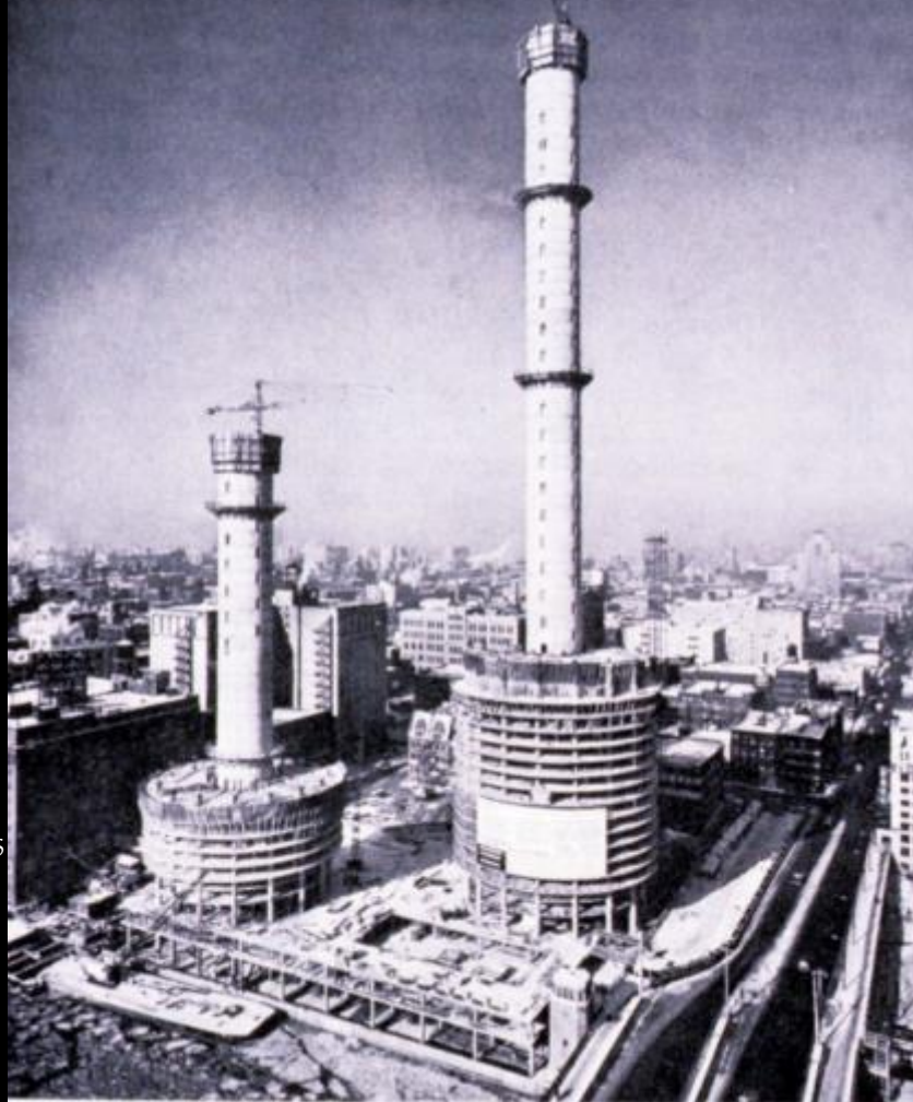
FIGURE 7.18 Marina Towers in Chicago during construction.
