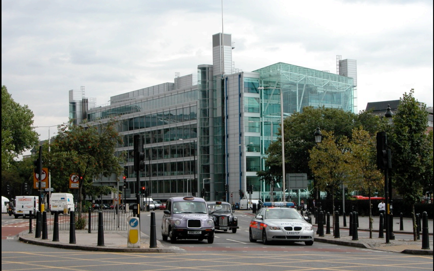
Tower Bridge House, London Richard Rogers
