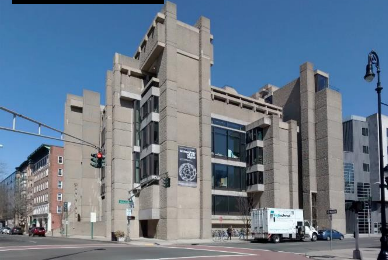
Yale Art and Architecture Building New Haven, CN Paul Rudolph 1963
