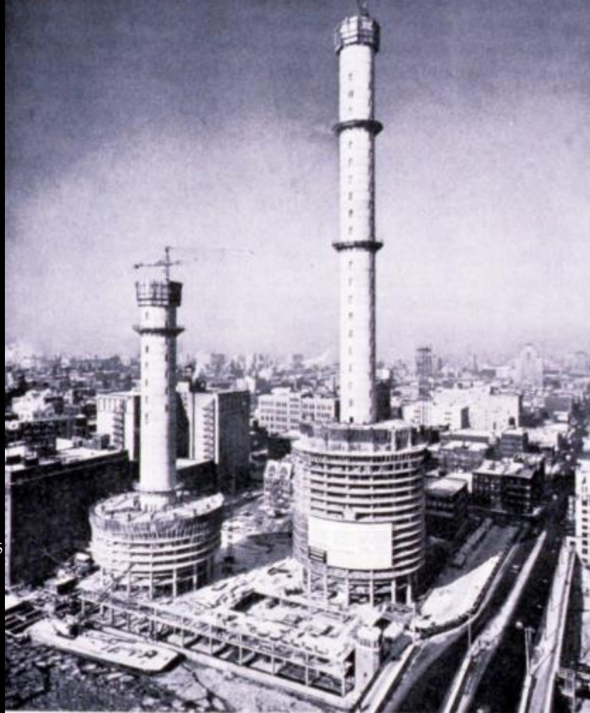
FIGURE 7.18 Marina Towers in Chicago during construction.
