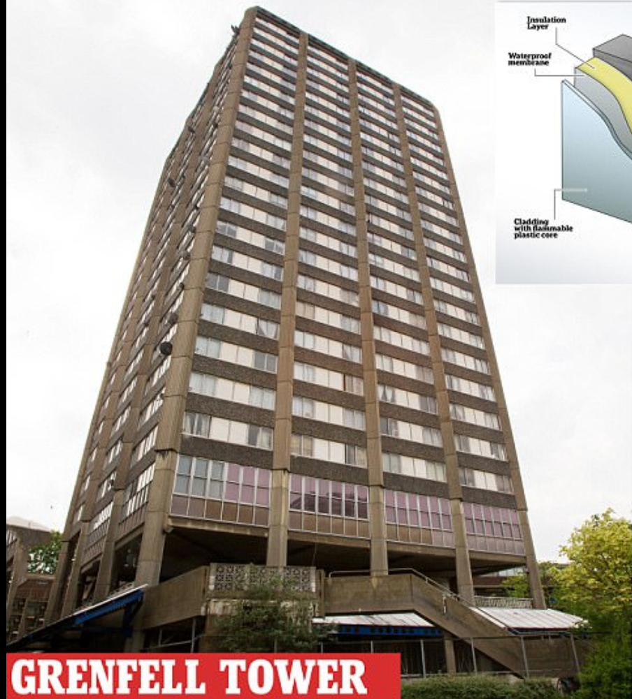
POST REFURB WITH NEW CLADDING
