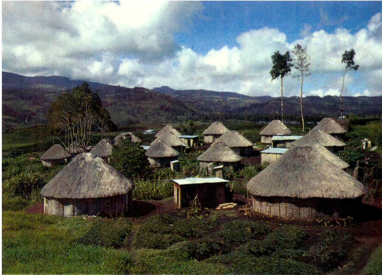
Conical thatched grass roofs top circular dwellings built with interlaced fiber siding , Village in New Guinea
