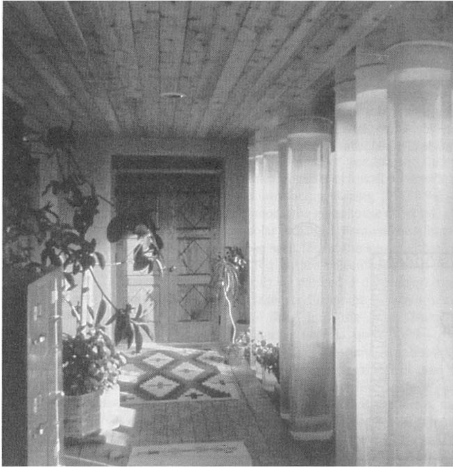
Figure 7.9d A Trombe wall can consist of vertical tubes filled with water. The tubes can be opaque, translucent, or transparent. (Courtesy of and © Solar Components Corporation.)
