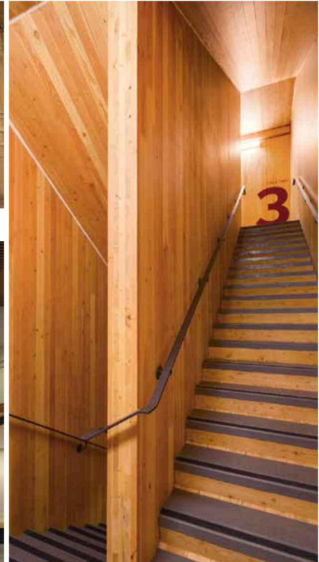
Stairwell with CLT walls, ceiling and floor
