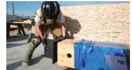
Installation of glulam column-to-column connector
