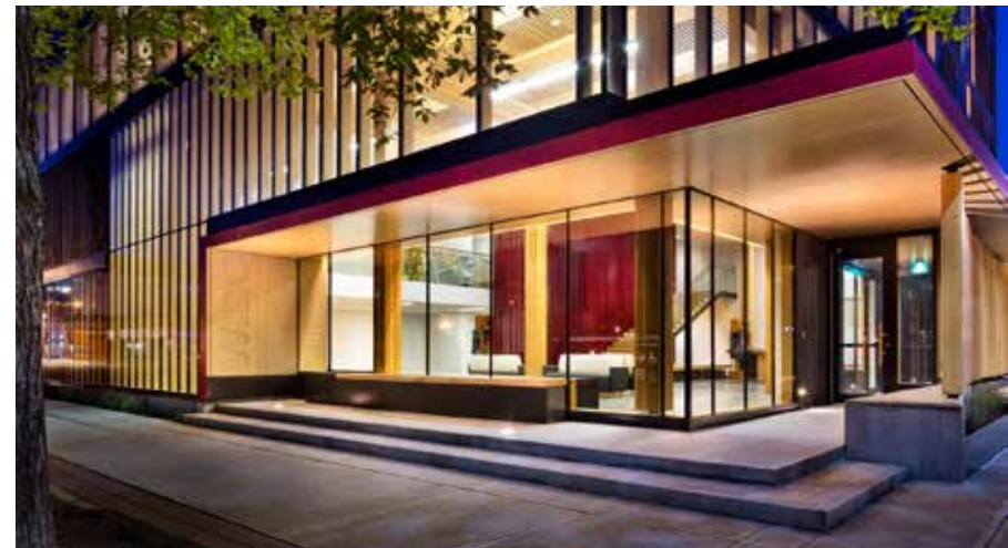
View of entrance
