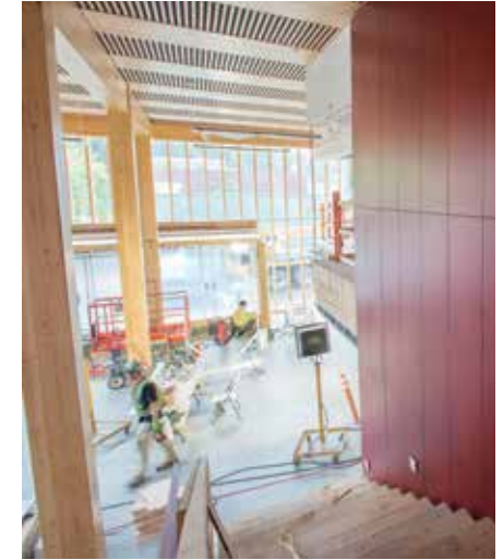
Red-stained plywood feature wall during construction
