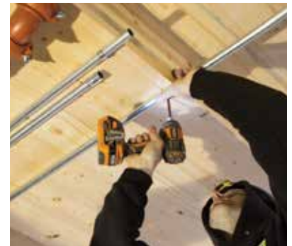
Installation of services below CLT floor
