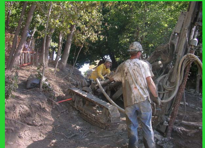
Difficult foundations for a tree, sloped site for the Grand House Student Cooperative in Cambridge, Ontario, Canada
