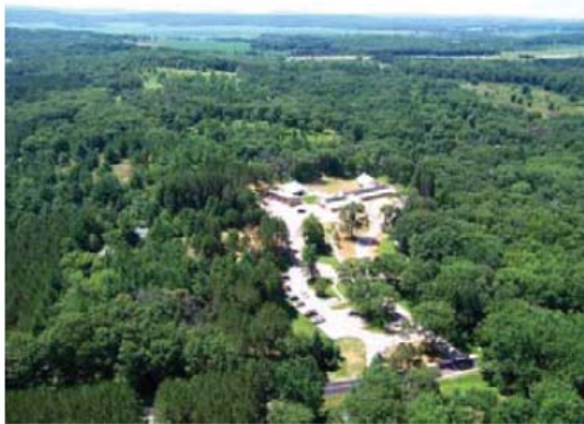
Aerial Image from South
