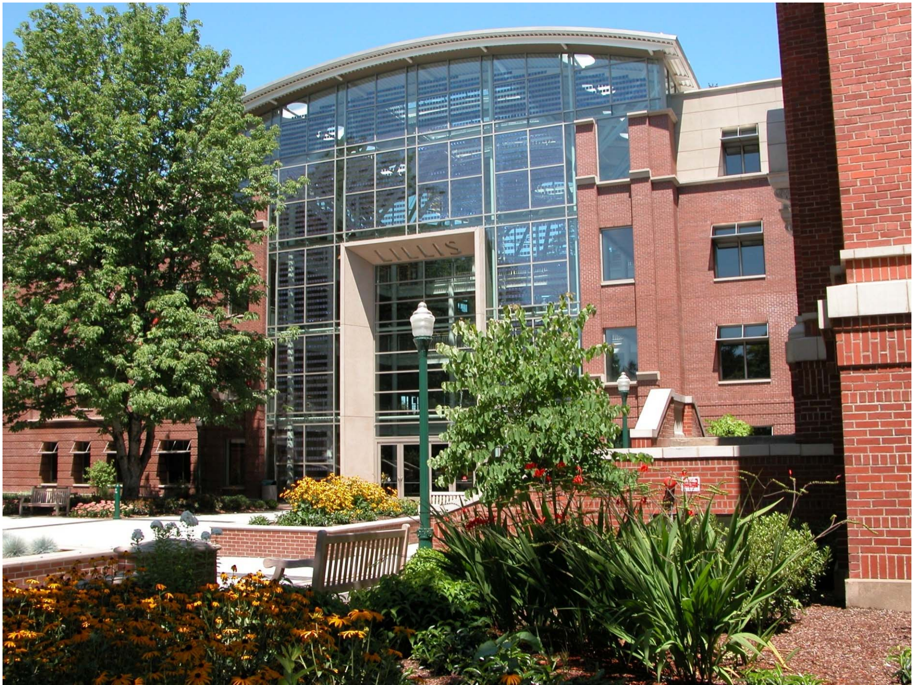
Thin PV integrated into the glazing at Lillis School of Business, U of Oregon
