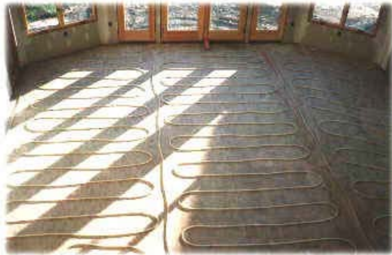
Step 1: The tubing is installed to the sub-floor of the home...
