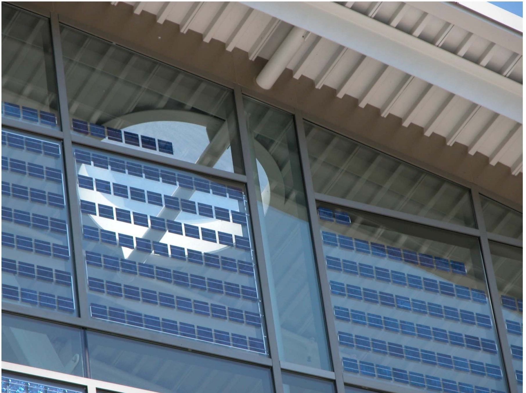
Thin PV integrated into the glazing at Lillis School of Business, U of Oregon
