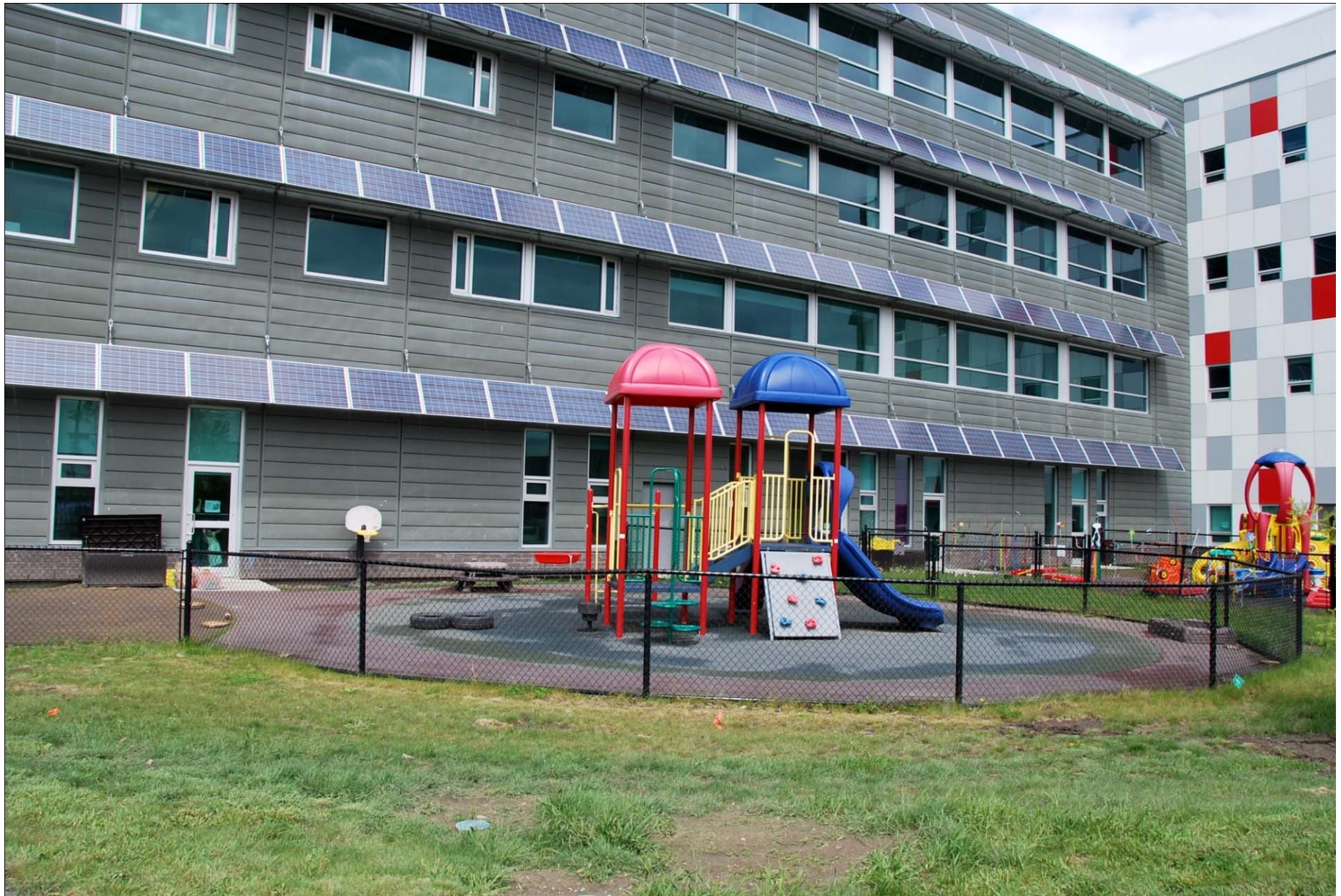
The PV on the Calgary Child Centre is used simultaneously as shading devices for the windows.
