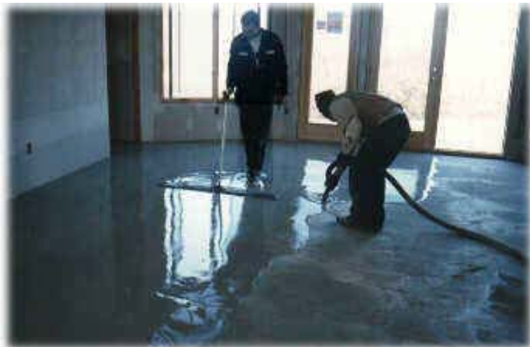
Step 4: The gypsum surface is smoothed to a glass-like finish & left to dry...
