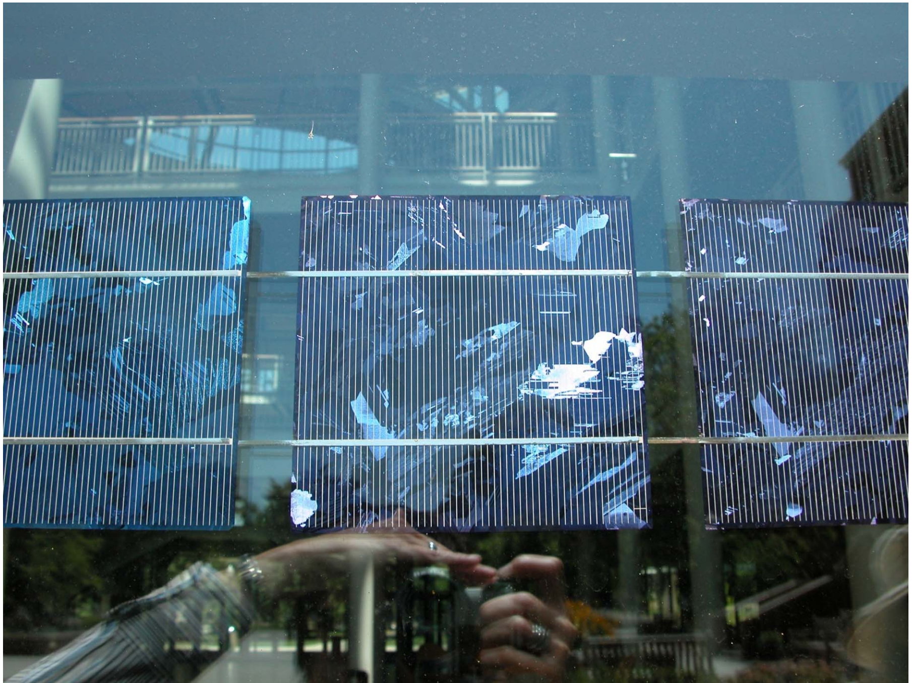
Thin PV integrated into the glazing at Lillis School of Business, U of Oregon
