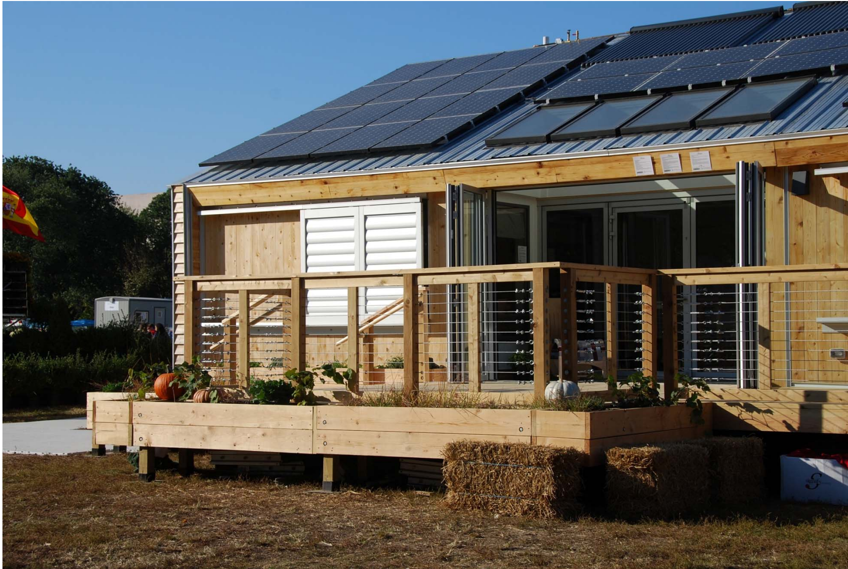
The glass doors at the center of Iowa's Solar Decathlon 2009 entry enclose a sun space.
