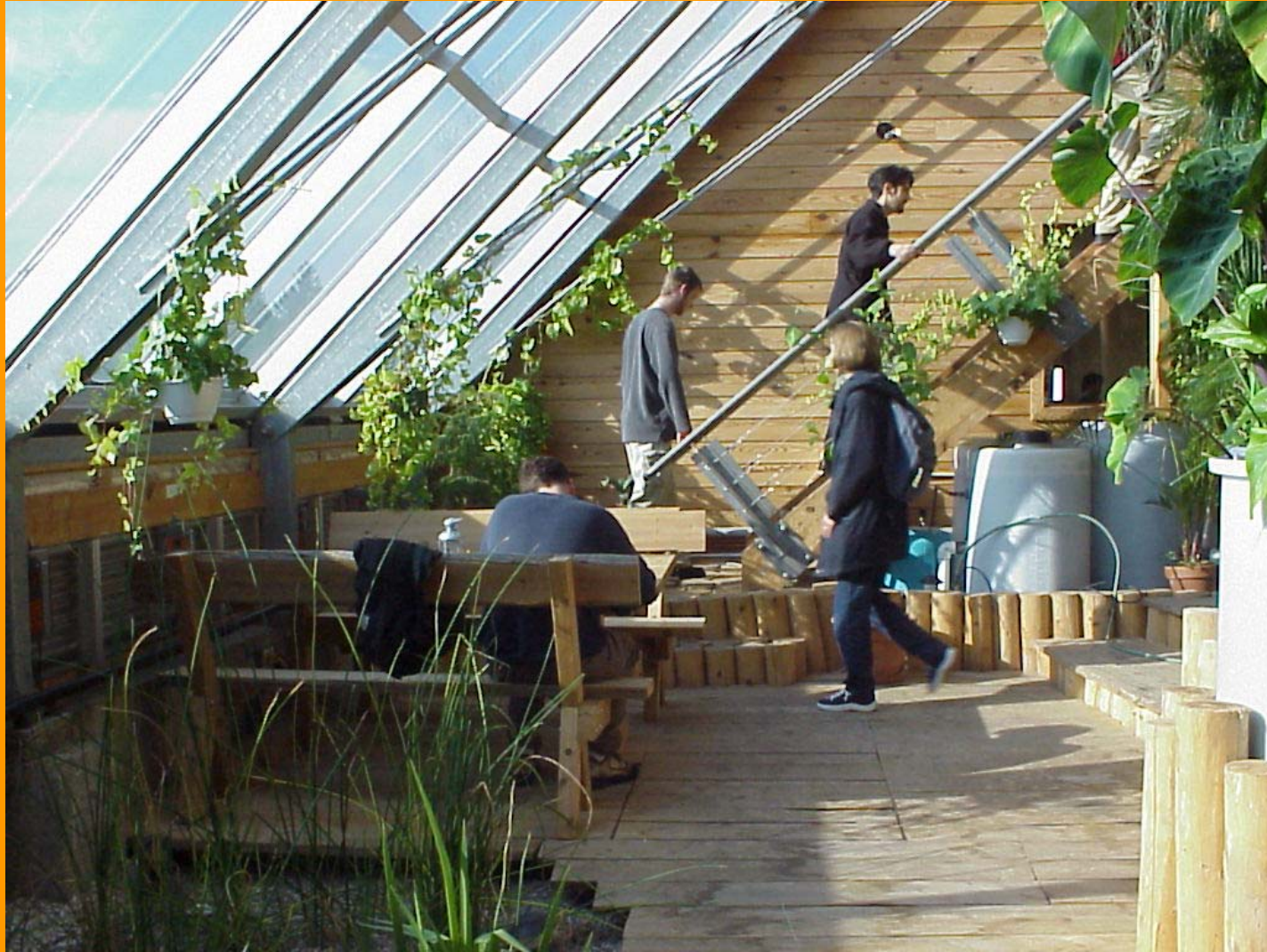
At the YMCA Solarium Building, the sunspace is used to house the Living Machine, and the heat caught in this space pumped to other portions of the building to heat them.
