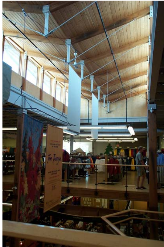
Mountain Equipment Coop, Ottawa
